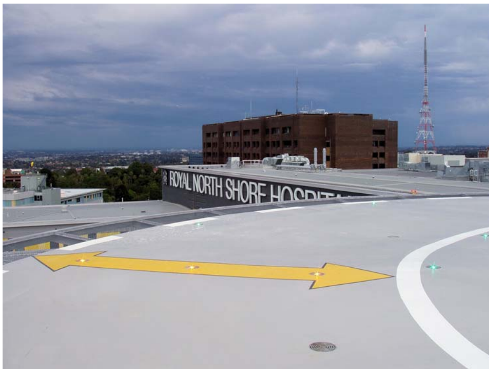
Figure 8: Approach/Departure Directional Arrow and Lights
