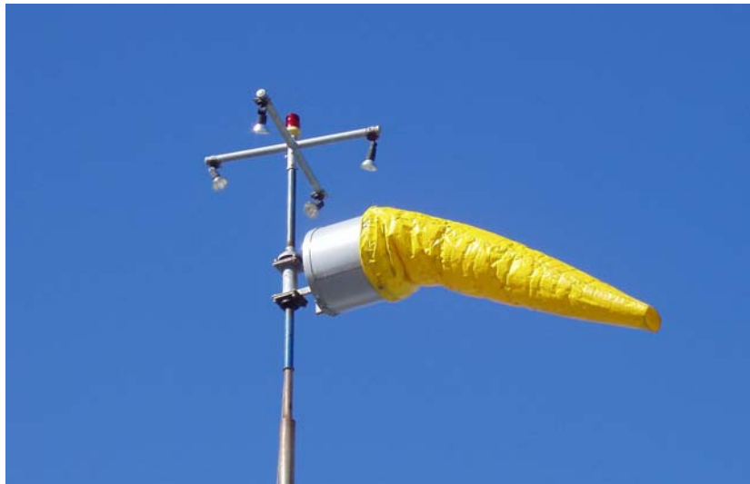
Figure 9: Windsock and Lighting
